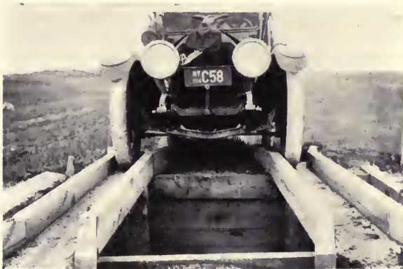
The Texas method of passing through wire fences without the use of gates. A most practical and timesaving device
